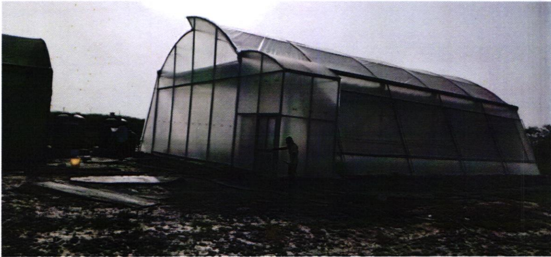
Fig:1 Polyhouse (250 sqm -25 x 10 ) naturally ventilated
