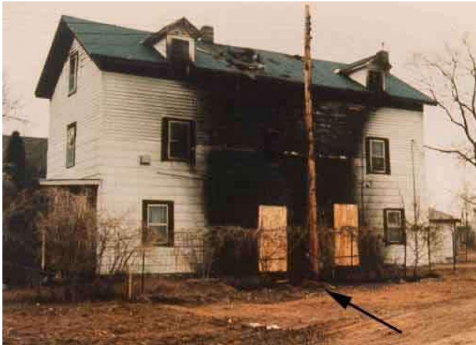
Figure 2: A photograph showing classic V pattern at origin of fire.
